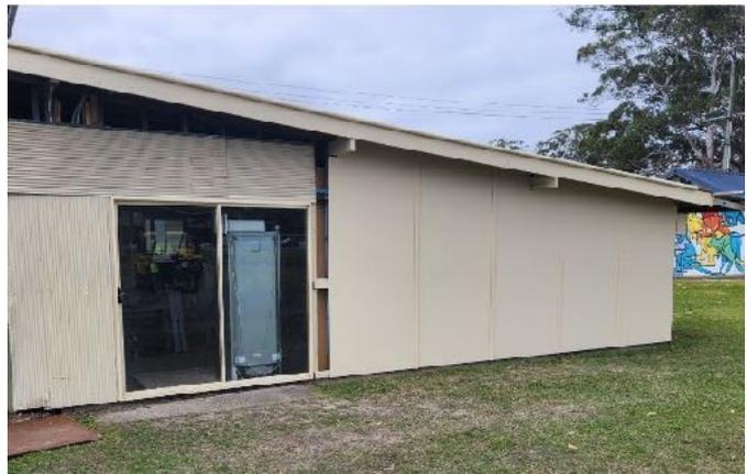
Above: You can see the progress on the facade: the mini orb sliding door has been replaced by a glass door and to the right of the glass door is now painted blue board, not mini orb. This makes the building more in keeping with the other buildings in the showground.
