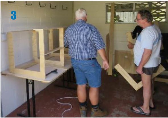
After the others arrived, we began making up one of the end modules. Both of the end modules have a solid piece of plywood on one end with a hole to allow the trains to enter and exit the layout where the tracks will connect to the fiddle yard.
