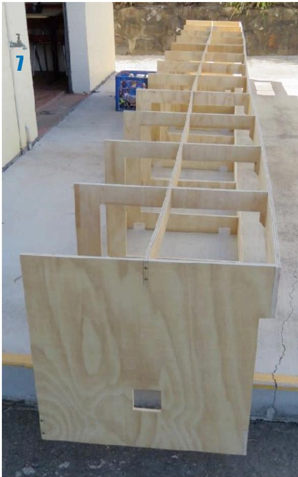
Also, I installed some brackets to strengthen the joint on the piece that I had damaged during the first working bee. The piece glued together successfully and didn't break during building.
