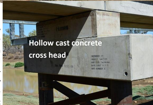
Hollow cast concrete cross head
