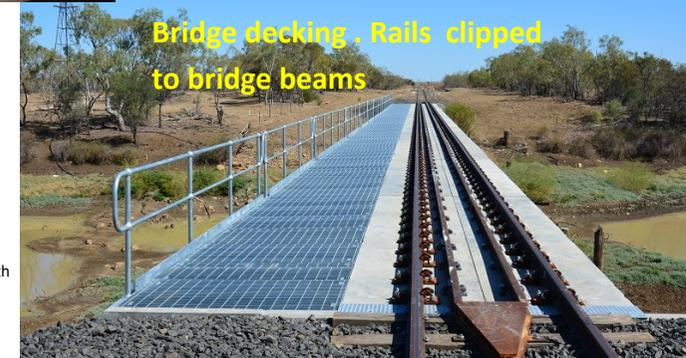
Bridge decking . Rails clipped to bridge beams
