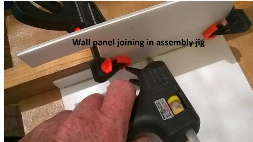
Wall panel joining in assembly jig
