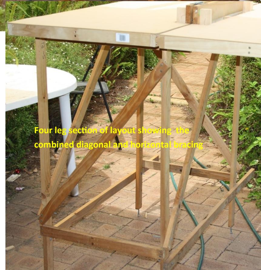
Four leg section of layout showing the combined diagonal and horizontal bracing
