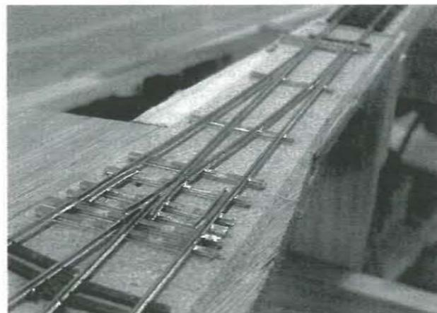
The track is pinned down every 100mm or so with 15mm x 1mm panel pins with their heads cut off - Ooooooh! Good metal straight edges are used for the straight bits and the usual easements are used on curves.
